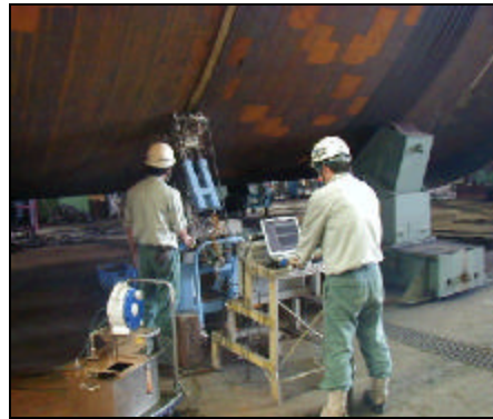
Post fabrication inspection using AUT system
