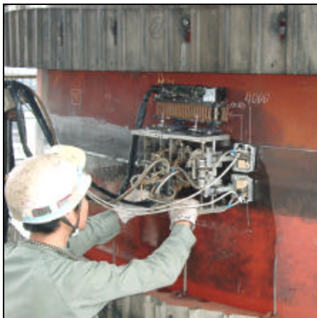
SEI personnel on-site with AUT equipment
