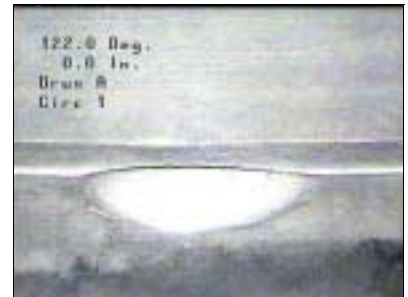
Cladding delamination as viewed from the video inspection and captured in digital form
