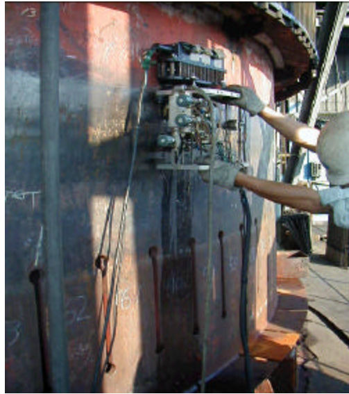
OUT OF SERVICE INSPECTION
